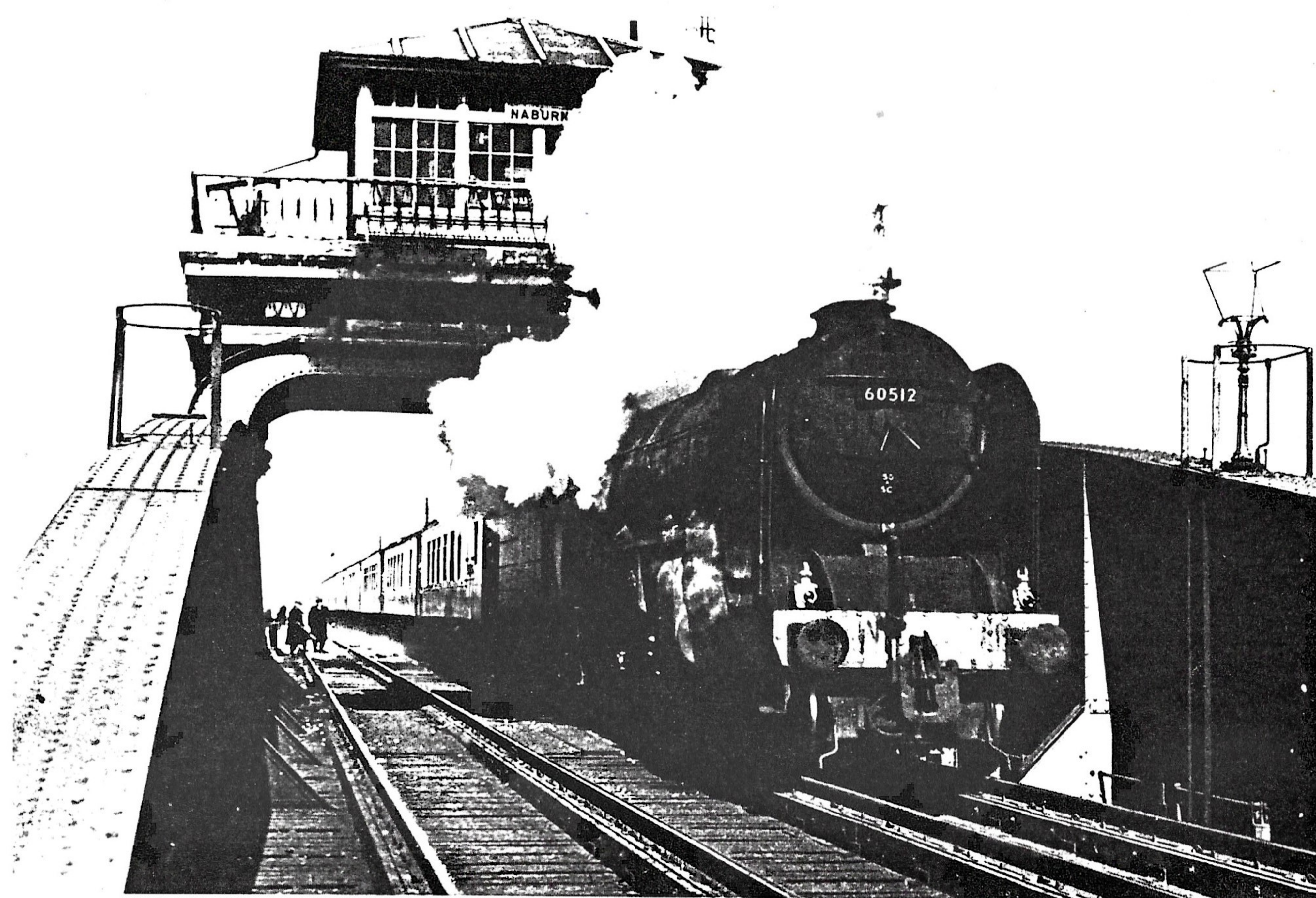
Just about everything in this mid-1950's picture has now gone. York A2/3 4-6-2 No. 60512 "Steady Aim" heads the up Tees-Tyne Pullman over Naburn Swing bridge which carried the York-Selby line over the River Ouse. The locomotive was scrapped in 1966, while the bridge became a fixed structure - the cabin aloft disappearing long before 1983 when the line itself was replaced by the East Coast main line diversion avoiding the new Selby coalfield.
